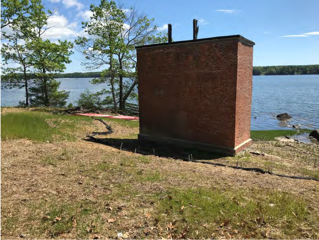
Fig 1: Slope leading down to cable house and salt marsh restoration at the west side of the bay. Viewing northeast. (05-24-21)
