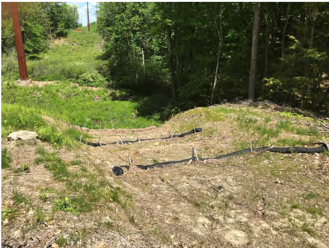
Fig 8: Lower portion of slope between Strs. 28 and 29. Viewing northeast. (05-24-21)
