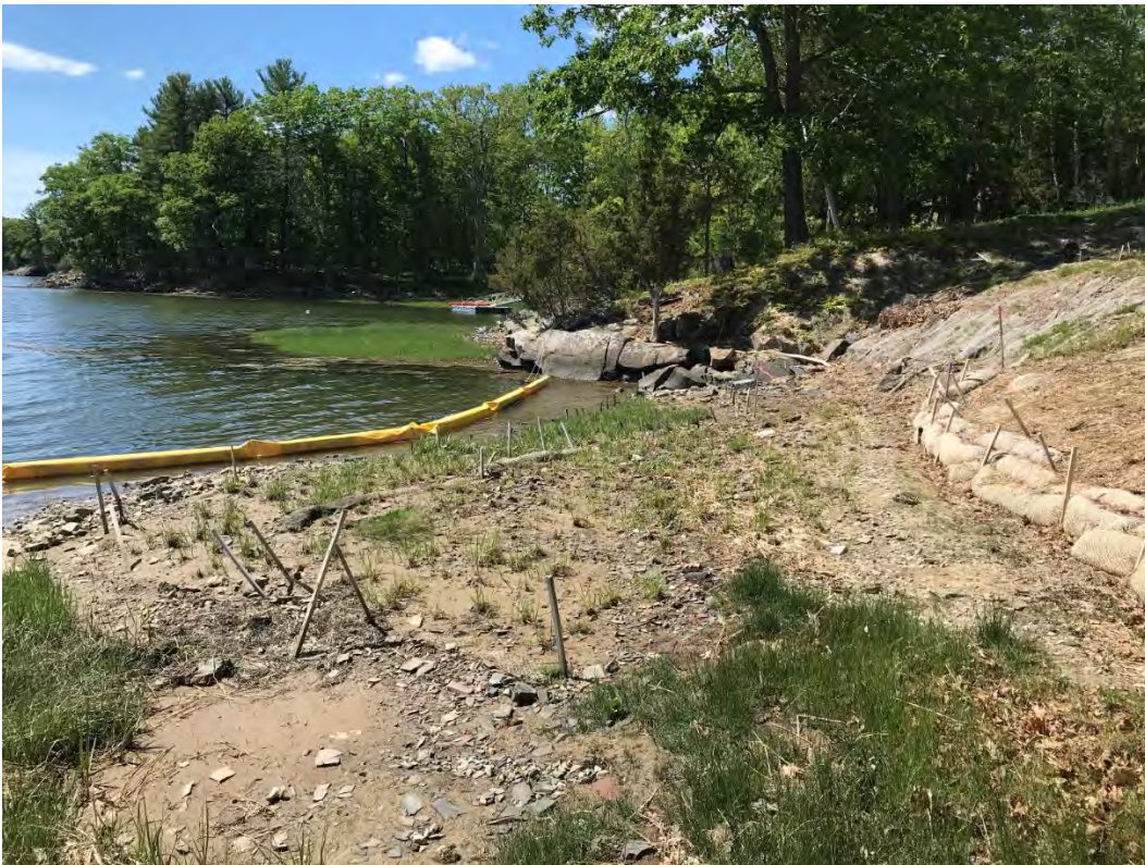
Fig 4: Toe of the slope and salt marsh restoration at the west side of the bay. Viewing south. (05-24-21)
