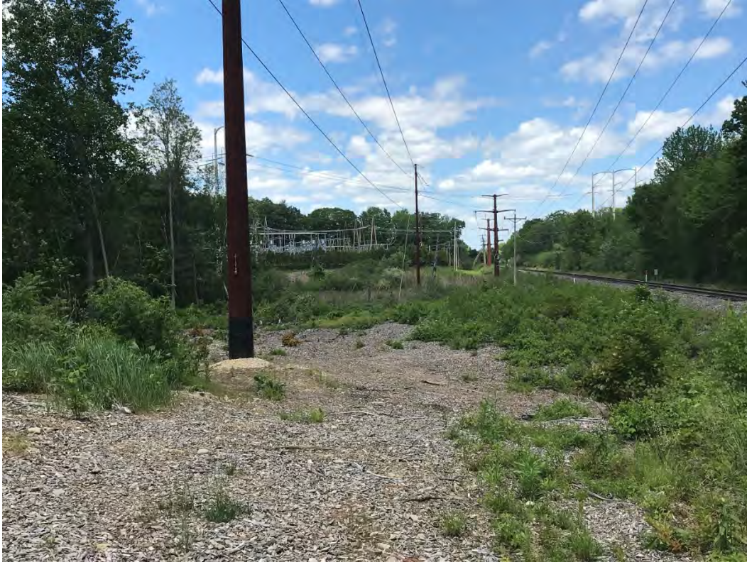
Fig 15: Str. 4 work area. Viewing north. (05-24-21)
