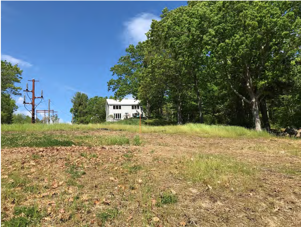
Fig 3: Slope above the cable house at the west side of the bay. Viewing northwest. (05-24-21)
