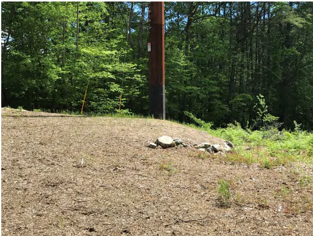
Fig 6: Str. 90 work area. Viewing northeast. (05-24-21)
