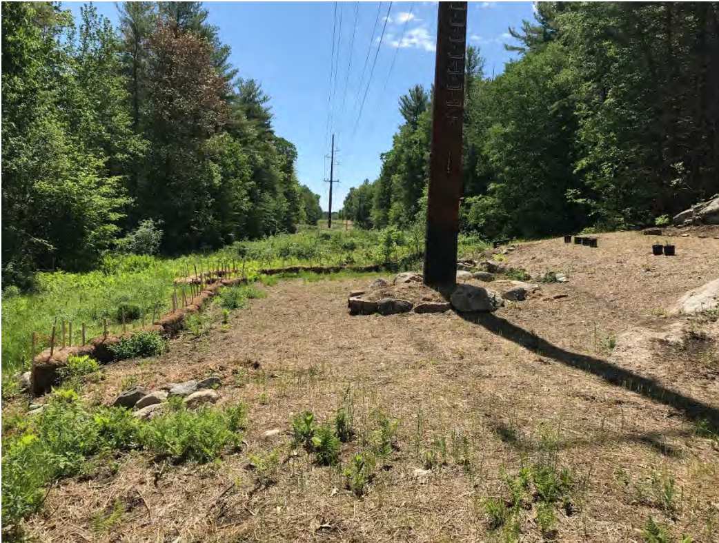
Fig 5: Str. 89 work area. Viewing southeast. (05-24-21)
